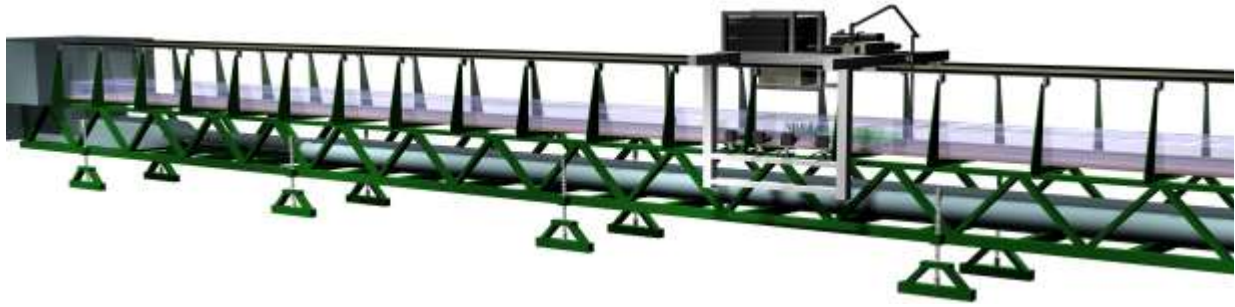
Figure 47. The Aberdeen Open Channel Facility (AOCF).
