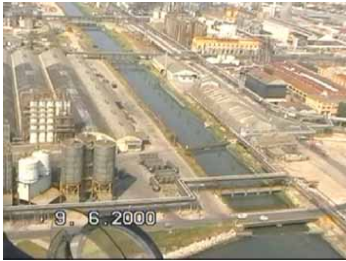
Figure 6.5: Lusore-Brentella channel within Porto Marghera petrochemical plant.
